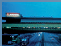
AUTOGRILL® BRIDGE CANTAGALLO, A1 MOTORWAY, BOLOGNA (ITALY)
