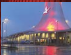
AUTOGRILL® VILLORESI EST, A8 MOTORWAY, MILANO (ITALY)
