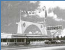
FIRST AUTOGRILL® PAVESI ON ITALIAN MOTORWAYS, A4 MOTORWAY, NOVARA (ITALY)
